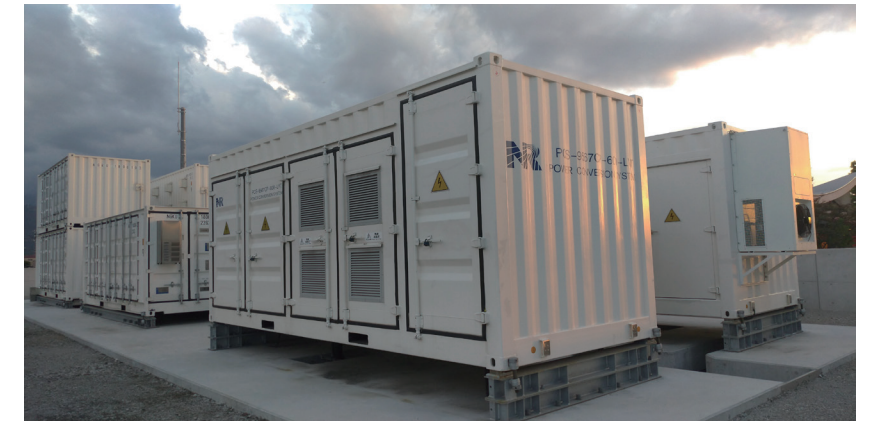
1.2MW/7.2MWh NGK Shikoku Island ITO sodium-sulfur battery energy storage project, Japan Peak shaving and valley filling, auxiliary frequency and voltage regulation
