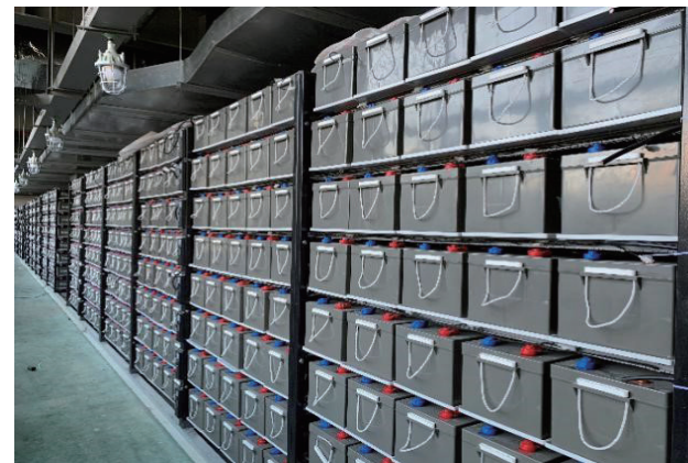
12MW/48MWh Jinling Station Lead-acid Battery Energy Storage Project Huzhou, Zhejiang
