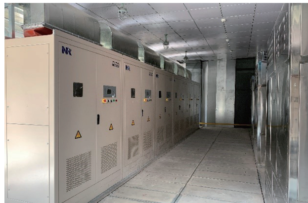
12MW/48MWh Jinling Station Lead-acid Battery Energy Storage Project Huzhou, Zhejiang
