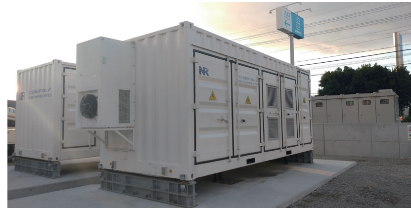
1.2MW/7.2MWh NGK Shikoku Island ITO sodium-sulfur battery energy storage project, Japan Peak shaving and valley filling, auxiliary frequency and voltage regulation
