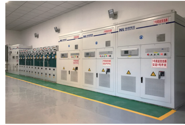
300kW/340kWh Low-voltage flexible distribution network lithium battery energy storage + DC distribution network converter project Xuzhou, Jiangsu
