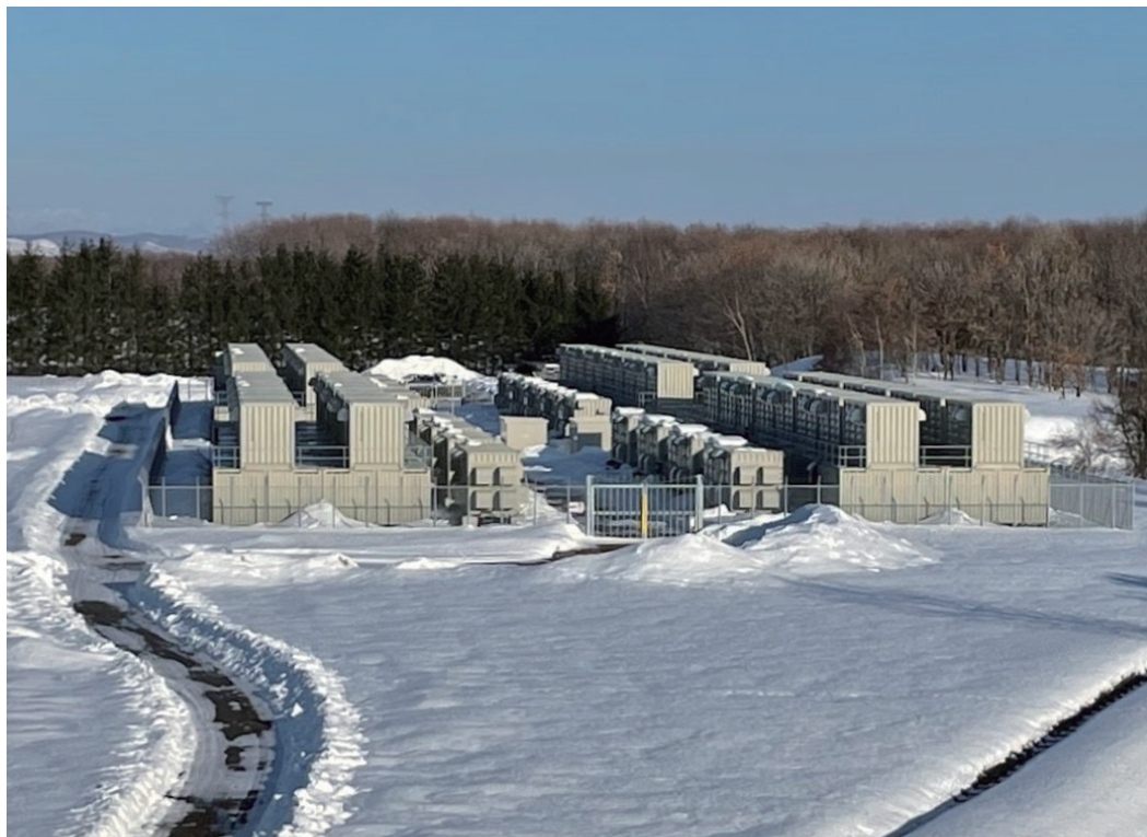
18MW/54MWh Hokkaido HEPCO Energy Storage Project, Japan Peak shaving and valley filling, auxiliary frequency regulation
